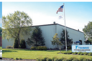
UST Sandusky Plant
