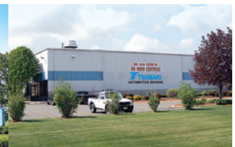
UST Chicopee Plant
